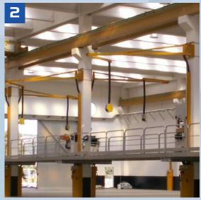
At the same time, the B5 is often used also in more complex installations, in centralized systems (2). Using our article LT, this product is connected to big vacuum-cleaning centrals units designed to cover big areas.
