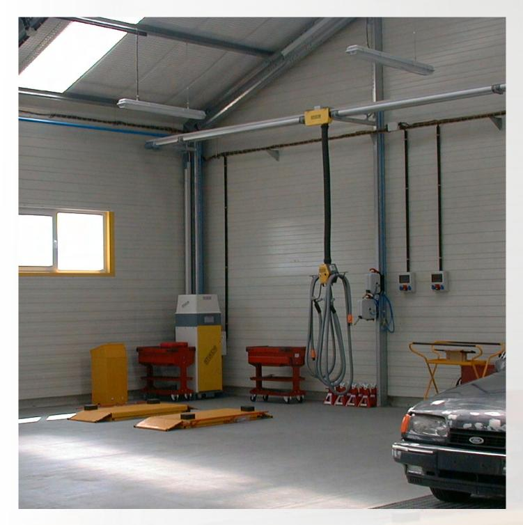
Exhausters with an high-performance sleeve – filtering system, a cleaning-filter system automatic and programmable and a control panel "touch screen" that allows to monitor the functioning and regulate the cleaning ranges. High energy-saving guaranteed by a switching-on / off automatic system that starts the suction turbine in the moment when the first-tool starts and stops it a few seconds after the switching-off of the last tool.
